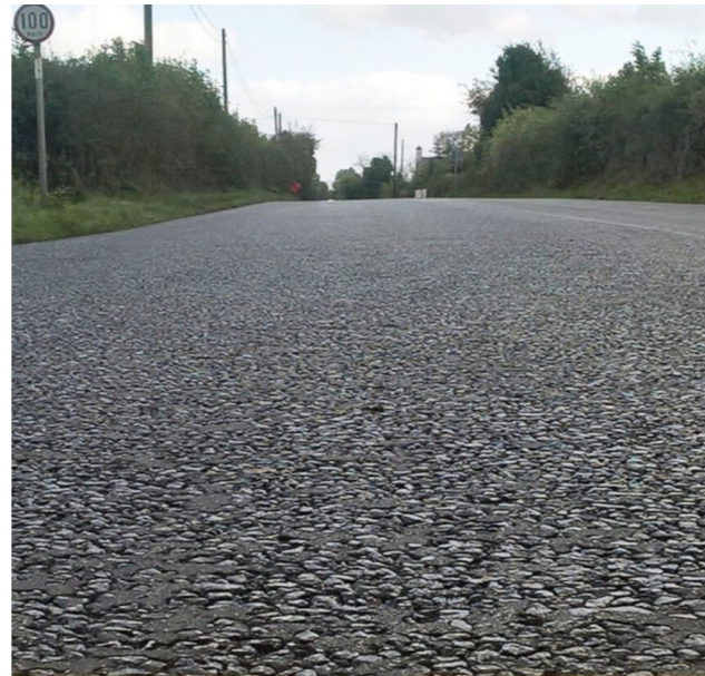
Asphalt to carriageway
